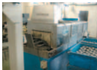
■Blow drying with compressed air (before improvements)
