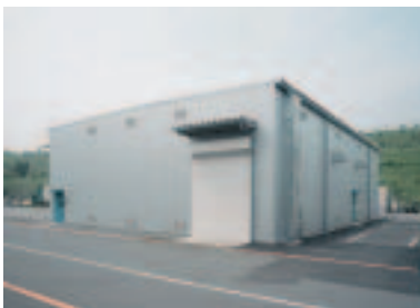
■ Next-generation, energy-conserving commercial store systems test facility A facility for developing fluorochemical-free, energy-conserving systems for freezing, refrigerating, and air conditioning
